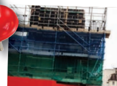
Brooklyn Court – completion due for Aug. 2015
