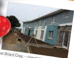
Ernest Briard Cres. – completion due for Jan. 2015
