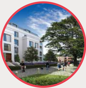
Summerland, St Helier No. of Properties: 82 homes Due for Completion: 2021
